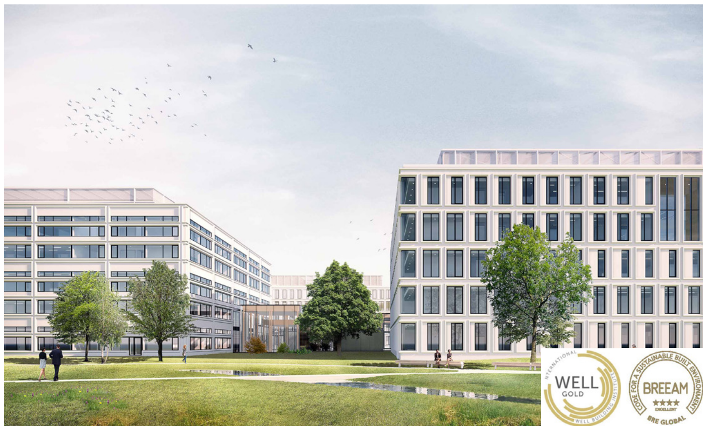
ASML De Run 1000: Architect EGM Architecten – foto: Norbert van Onna
